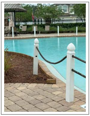
GMS staff removed old rope and caps from pool entry. Replaced with new rope, caps, and reset crooked post in 50lbs of concrete.
